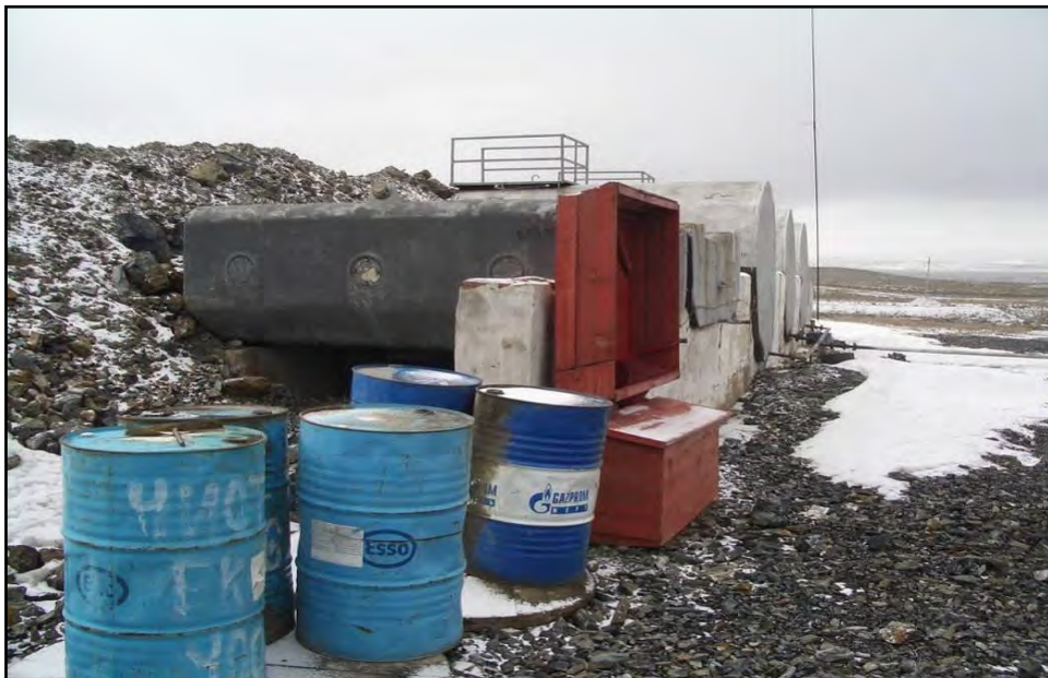
Figure 9-1: Fuel Drums (Foreground) and Tanks (Background) within Mine Waste Bund
